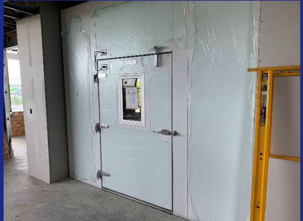
Cold Room - Second Floor
