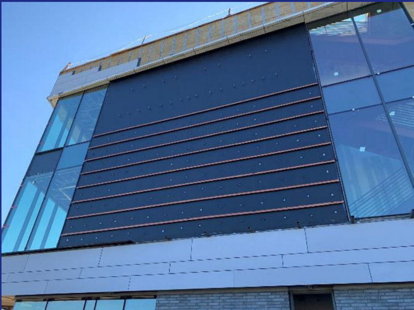
Preparing West side of building for signage
