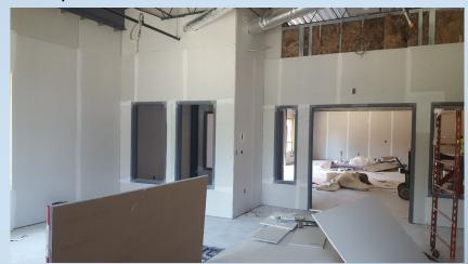
Sheetrock complete in all three sections, in process of installing windows. Started on IT rough in of data, digging footings retaining wall at rear of building.
